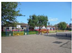
This playground is being refurbished over summer
